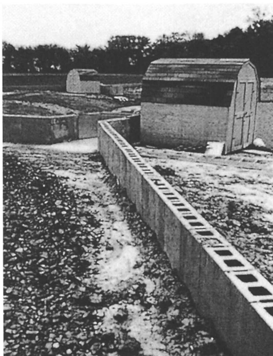
Figure 4. Concrete block retaining walls and primary flume sampling stations for quantifying runoff hydrology, sediment yield, and chlorpyrifos transport.
